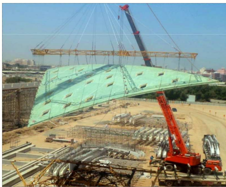
Completed: Al Haramain Railway Station KSA; 15.000 cbm; structural and thermal requirements (Foster)
