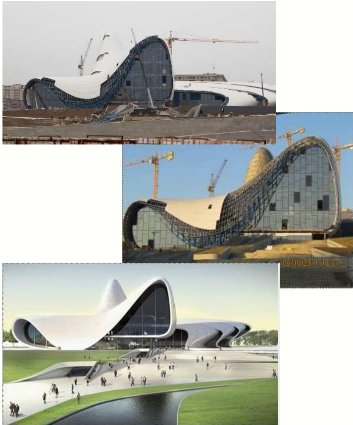
Haydar Aliyev Cultural Centre in Baku, Azerbaijan. 18,000m 2 panels; 50 yr building life span
