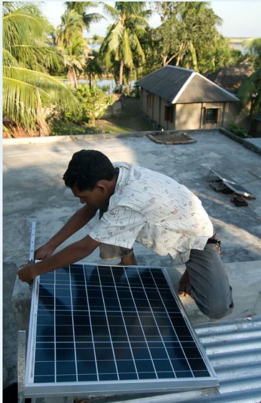
Installation eines Solar Home Systems in Bangladesch
