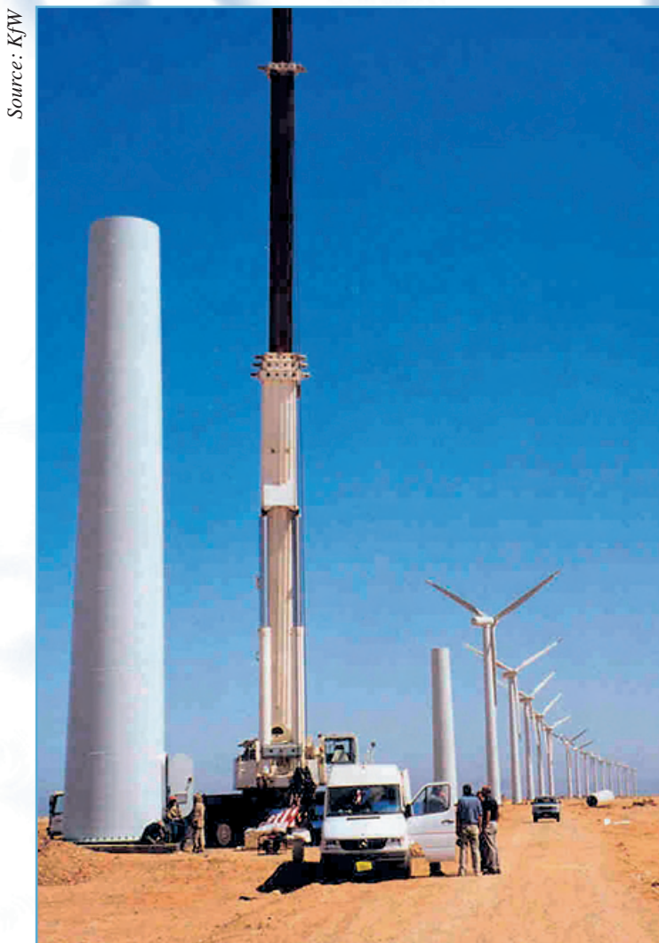
Constructing the Zaafarana wind farm, Egypt
