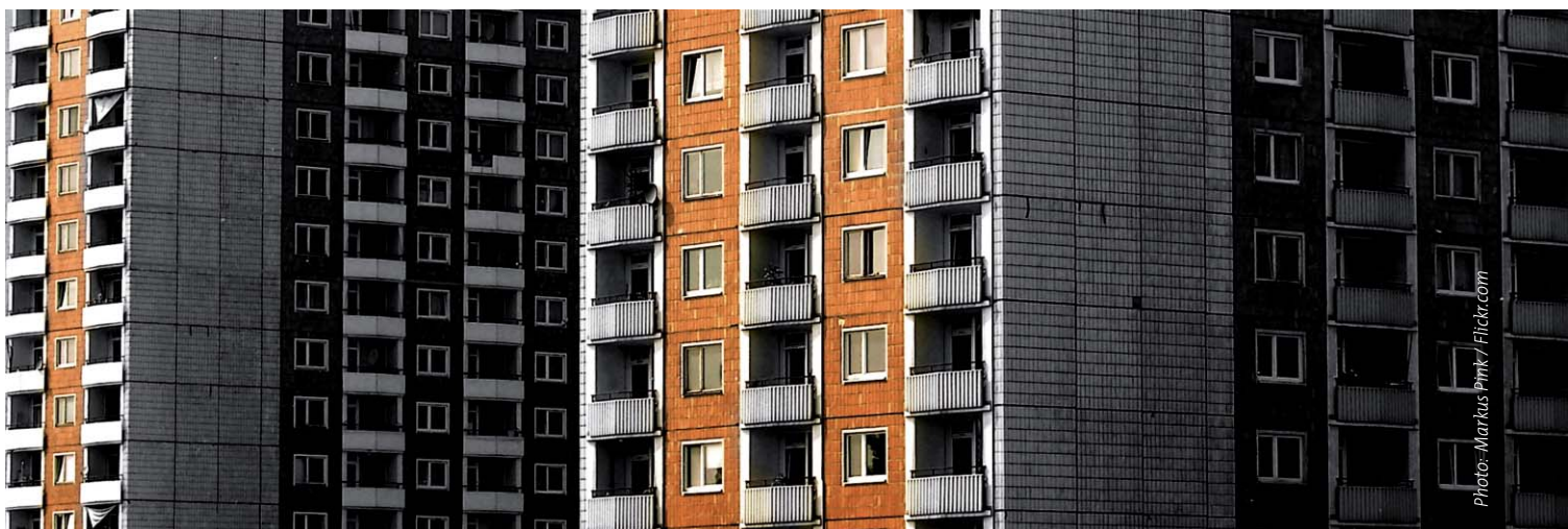
East-West Divide: Market mechanisms can assist the transfer of efficient technology. Huge potential is seen in the construction industries in Eastern and Central Europe.
