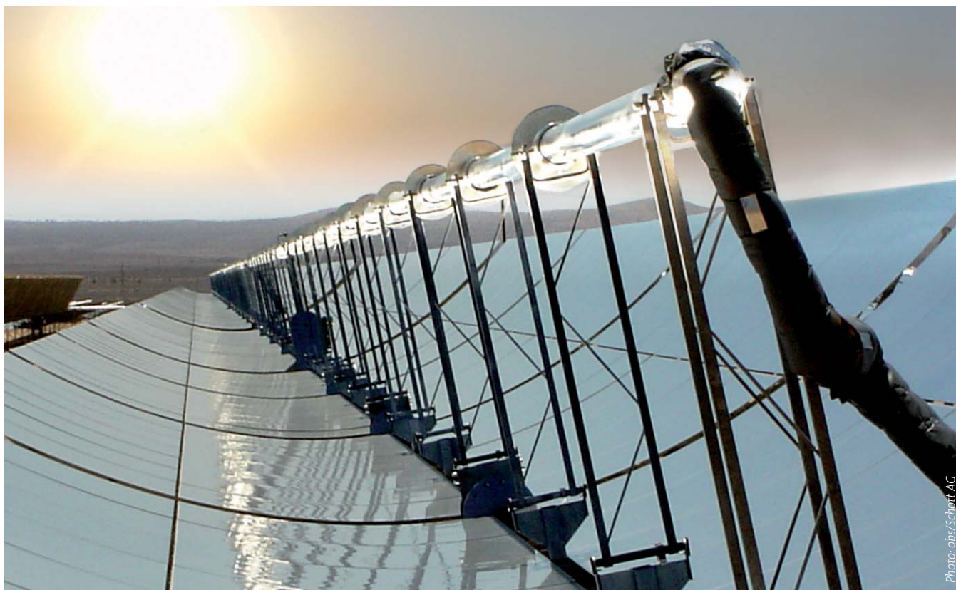
Role model EU: Parabolic trough technology used in large-scale solar power production
